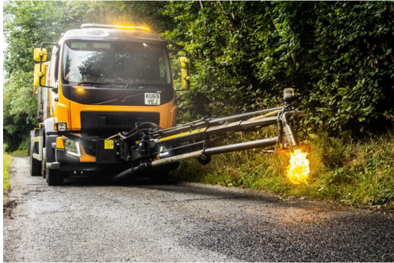
Fig. 1.13: Dragon patcher in operation.
