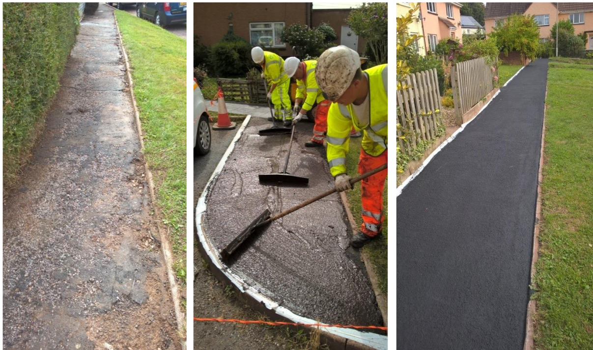
Fig. 2.8: Slurry seal being applied to a footway (Before, During and After)
