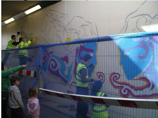
During – note public protection works
